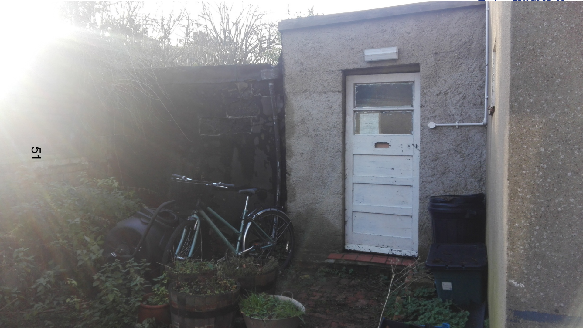
Rear of the site looking east
